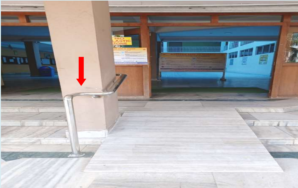
Figure 1: Ramp at Edu Building 1
