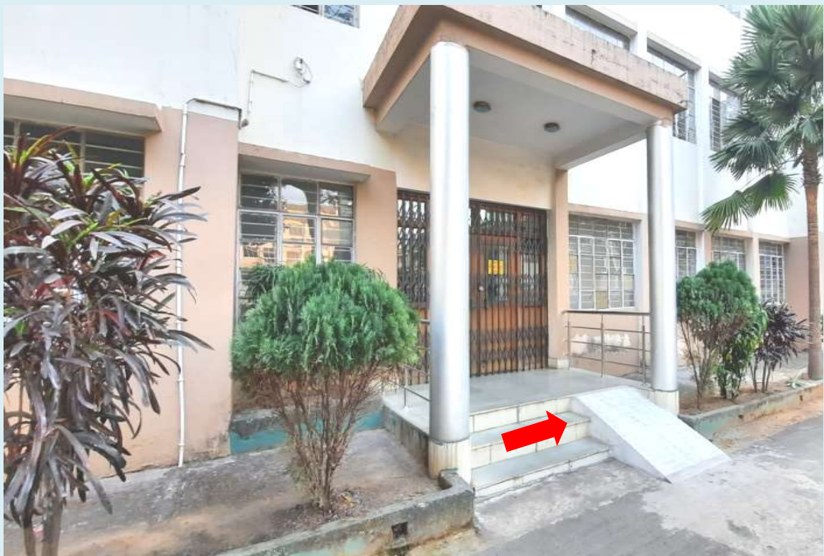
Figure 2: Ramp at Edu Building 2
