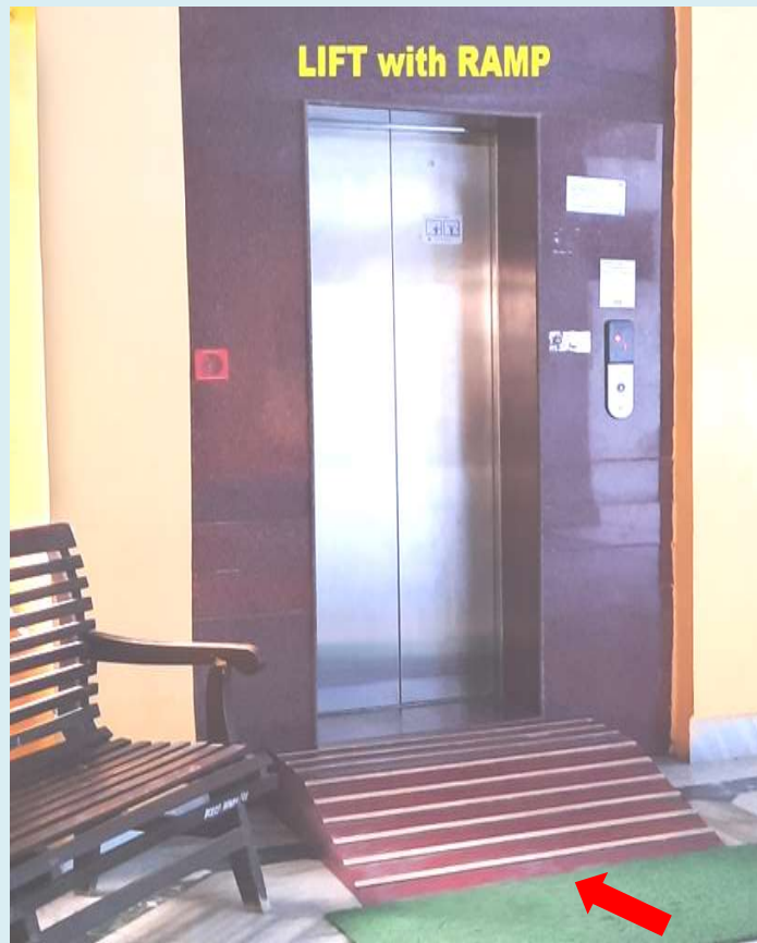
Figure 3: Lift with Ramp
